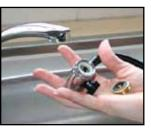
**Step 4. Determine Threads** A female faucet has threads on the inside. A male faucet has visible threads on the outside.
