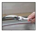
**Step 1. Remove Aerator** Unscrew the faucet aerator using your hand or a small tool such as pliers or a wrench.
