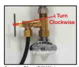
Step 1. Shut Off Water Undersink Only. Close the Shut-Off Valve by turning the handle clockwise.
