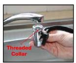
Step 5b: All Faucets Connect the diverter to the male faucet or adaptor by turning the threaded collar on the top of the diverter
