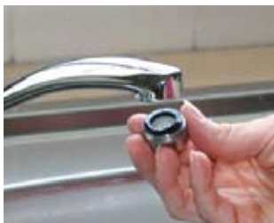
Step 2. Retain Washer The aerator & washers may be needed later. Set these pieces aside for safe-keeping.
