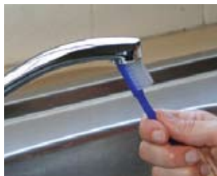
Step 3. Cleaning Clean the spout threads. To remove dirt, use an old toothbrush and flush with water.
