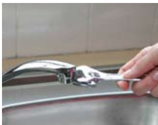
Step 1. Remove Aerator Unscrew the faucet aerator using your hand or a small tool such as pliers or a wrench.
