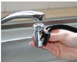
Step 5a. Male Faucet Determine thread type. A male faucet has visible thread on the outside . A female faucet has its thread on the inside .
