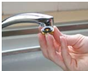
Step 5b. Female Faucet Attach the brass accessory to the spout. You may need a pair of pliers to tighten. DO NOT OVERTIGHTEN!
