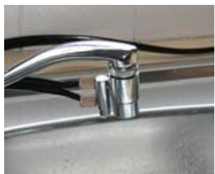
Step 6. Attach the adaptor. Screw down the locking nut till it is finger tight.
