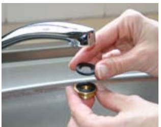
Optional: The brass accessory may require an extra washer to fit some spouts. Use the washer from the recently removed aerator (Step 2) if needed.
