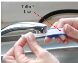
Handy Hint: In some cases, plumbers Teflon® tape (supplied) may be needed to achieve a water-tight seal for the brass accessory.
